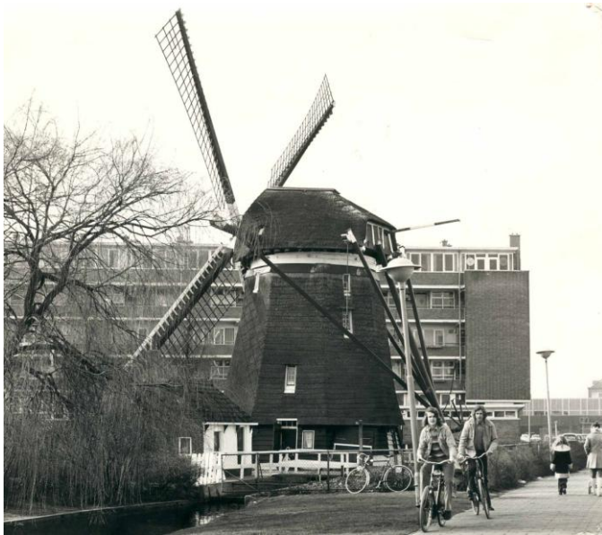
This is a picture of mill 'De Vlieger' at its old place near the Badhuislaan. You can see that flats have already been built near to the mill. Because of this the mill didn't get sufficient wind to turn properly.
